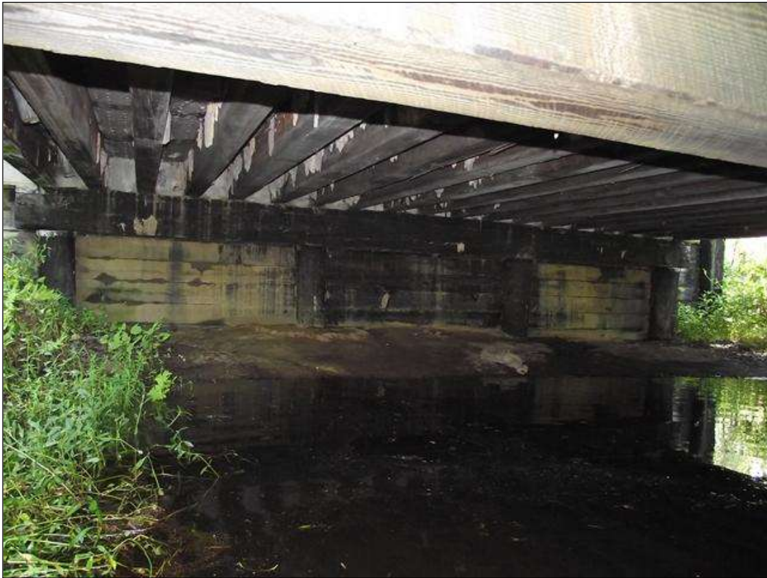
END BENT 2 OVERVIEW
