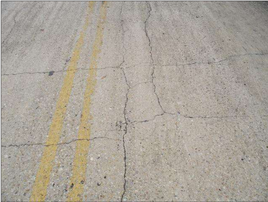
LONGITUDINAL AND TRANSVERSE CRACKING IN SPAN 1
