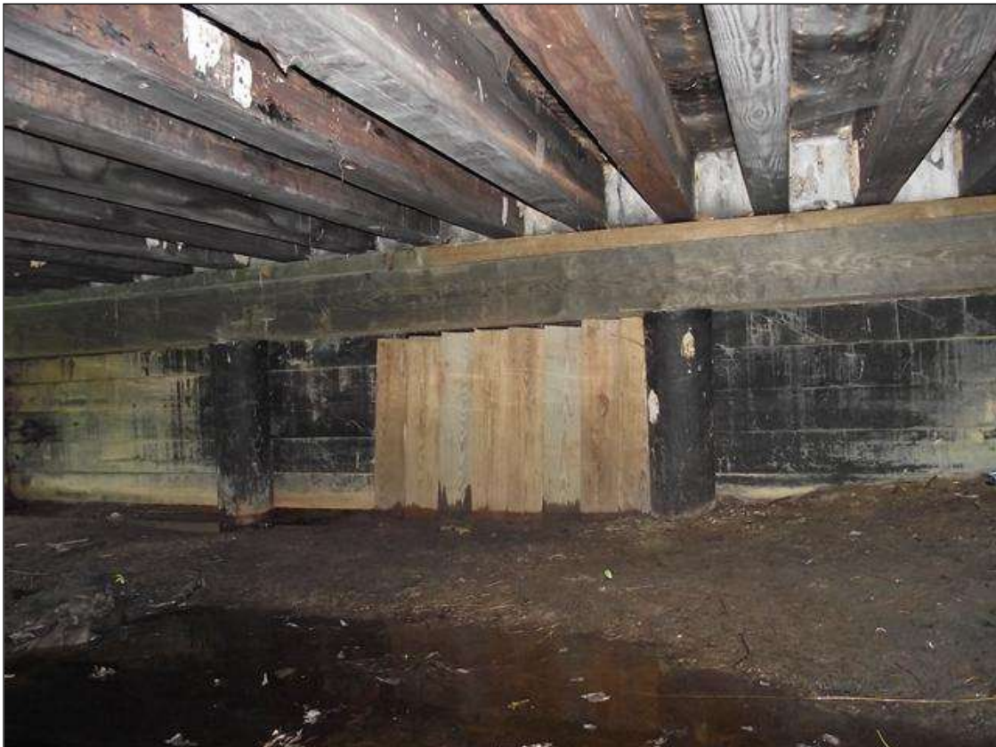
VERTICAL BOARDS FACE NAILED BETWEEN PILE 2 & 3 AT END BENT 1 BULKHEAD
