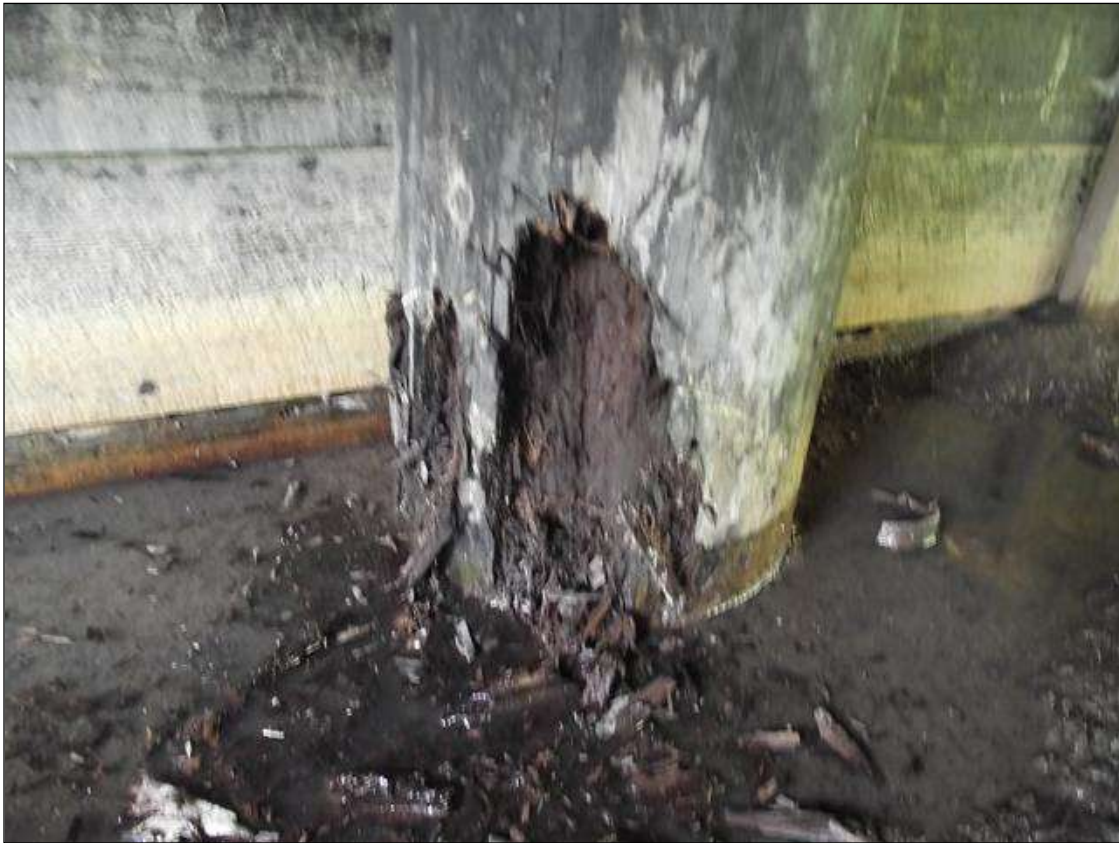
DECAY IN THE RIGHT SIDE OF PILE 3 AT END BENT 1 (PRIORITY MAINTENANCE ISSUED)
