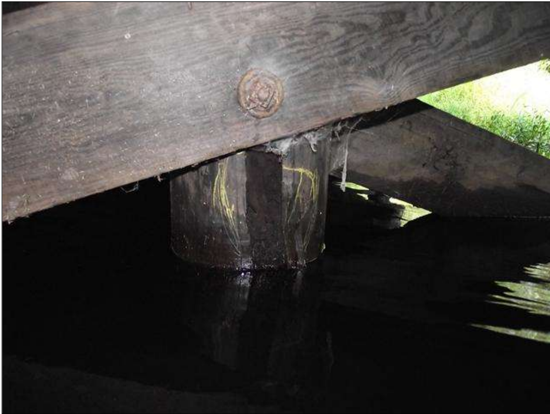
DELAMINATION IN PILE 2 AT BENT 2 SPAN 3 SIDE BELOW CROSSBRACE CONNECTION
