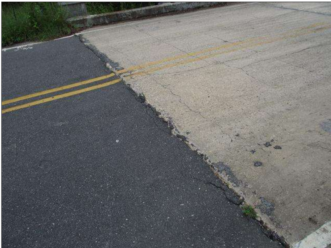
JOINT AT END BENT 1
