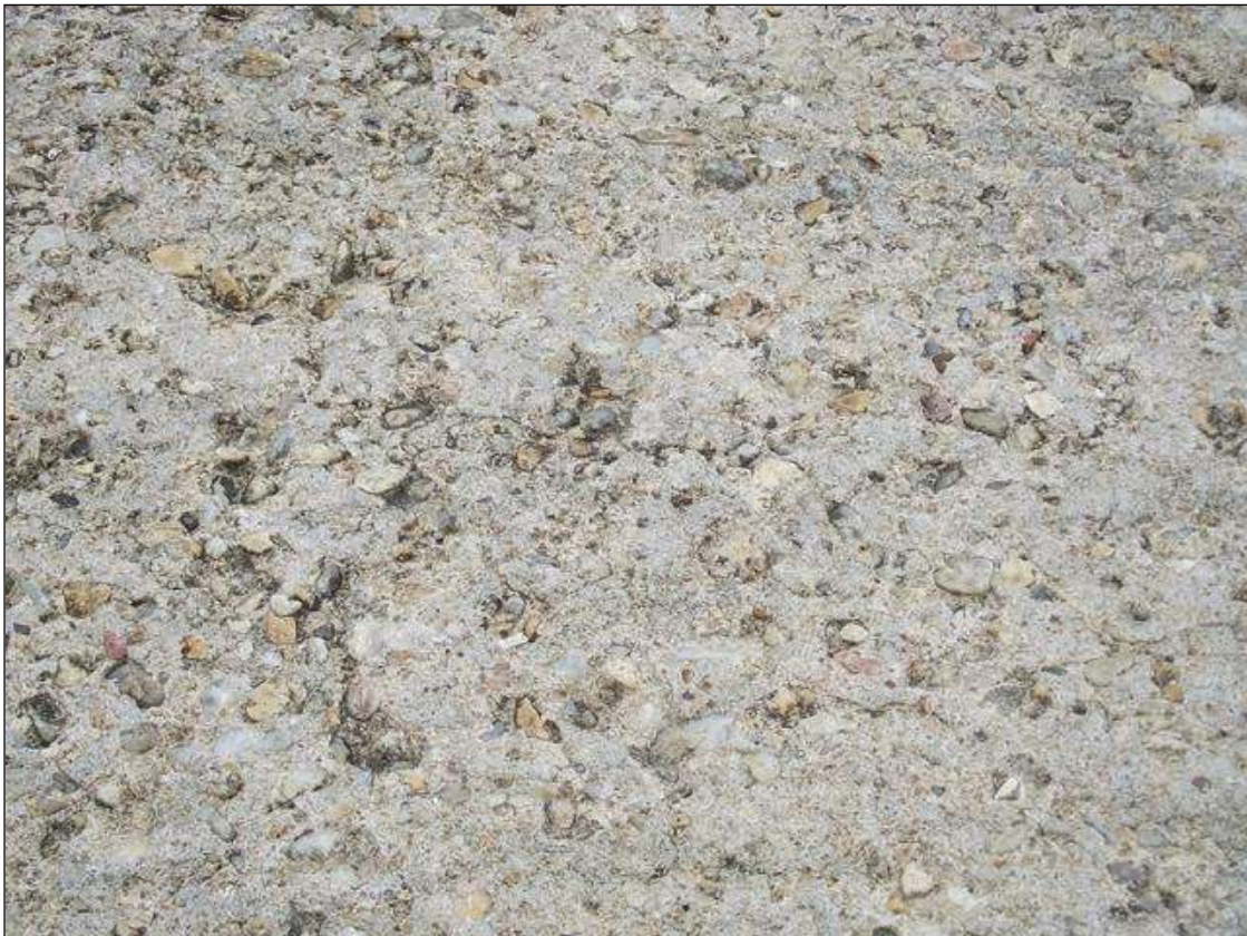
TOP OF DECK SCALED WITH EXPOSED AGGREGATE
