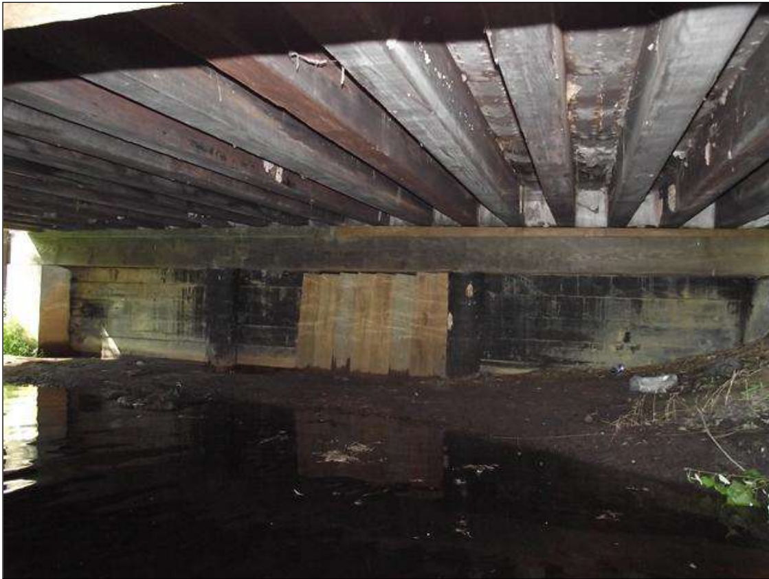
END BENT 1 OVERVIEW
