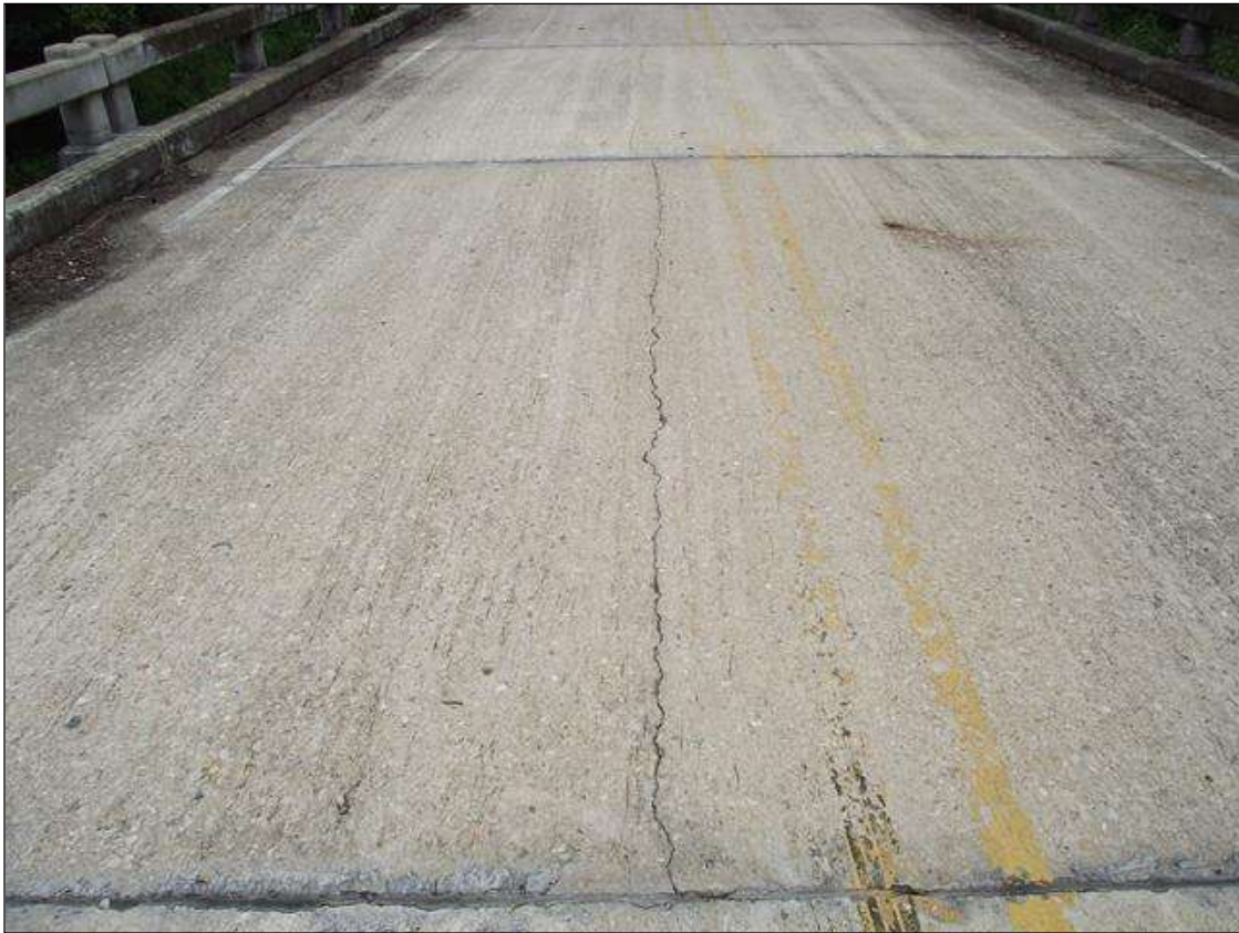
LONGITUDINAL CRACK IN SPAN 3, SIMILAR IN SPAN 2, 4 & 5
