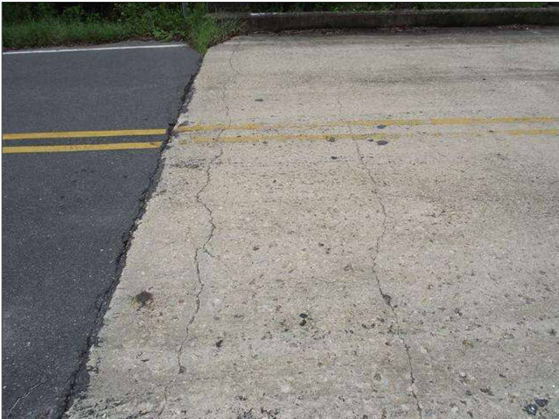
TRANSVERSE CRACKING IN SPAN 5
