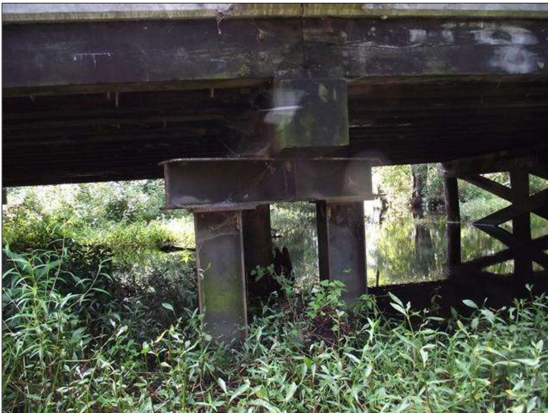
CRUTCH PILES AT BENT 3 LEFT END OF CAP
