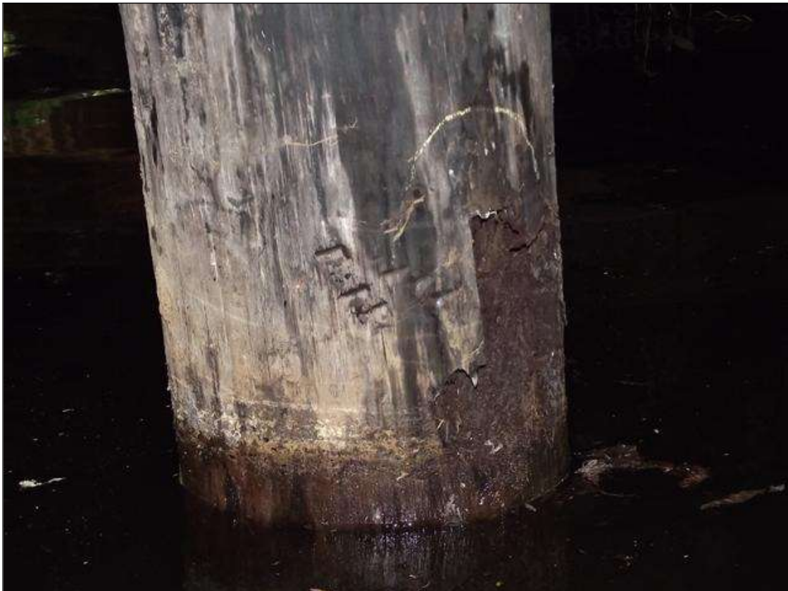
DECAY IN THE LEFT SIDE OF PILE 2 AT BENT 4 (PRIORITY MAINTENANCE ISSUED)
