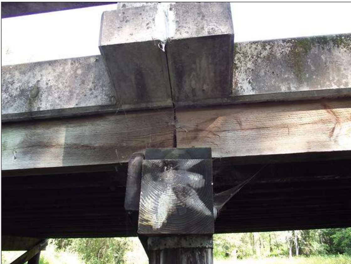
SUPERSTRUCTURE OVER END OF CAP
