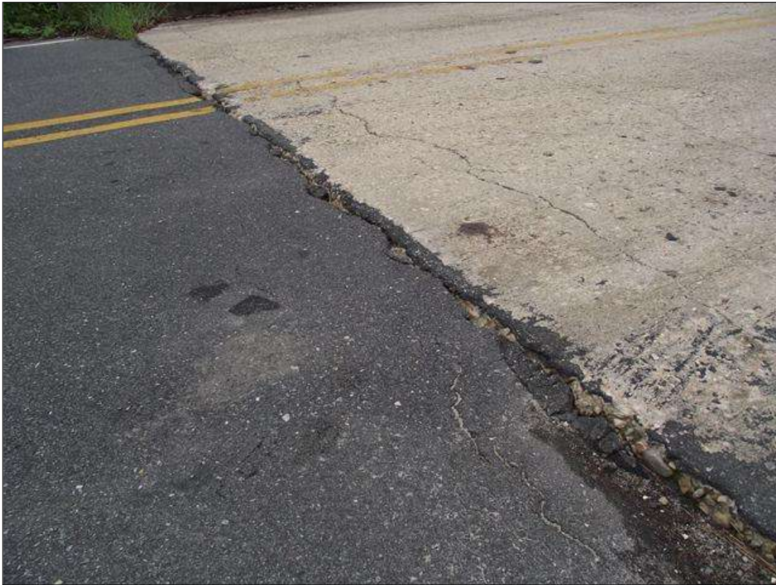
APPROACH 2 SETTLED AT END BENT 2
