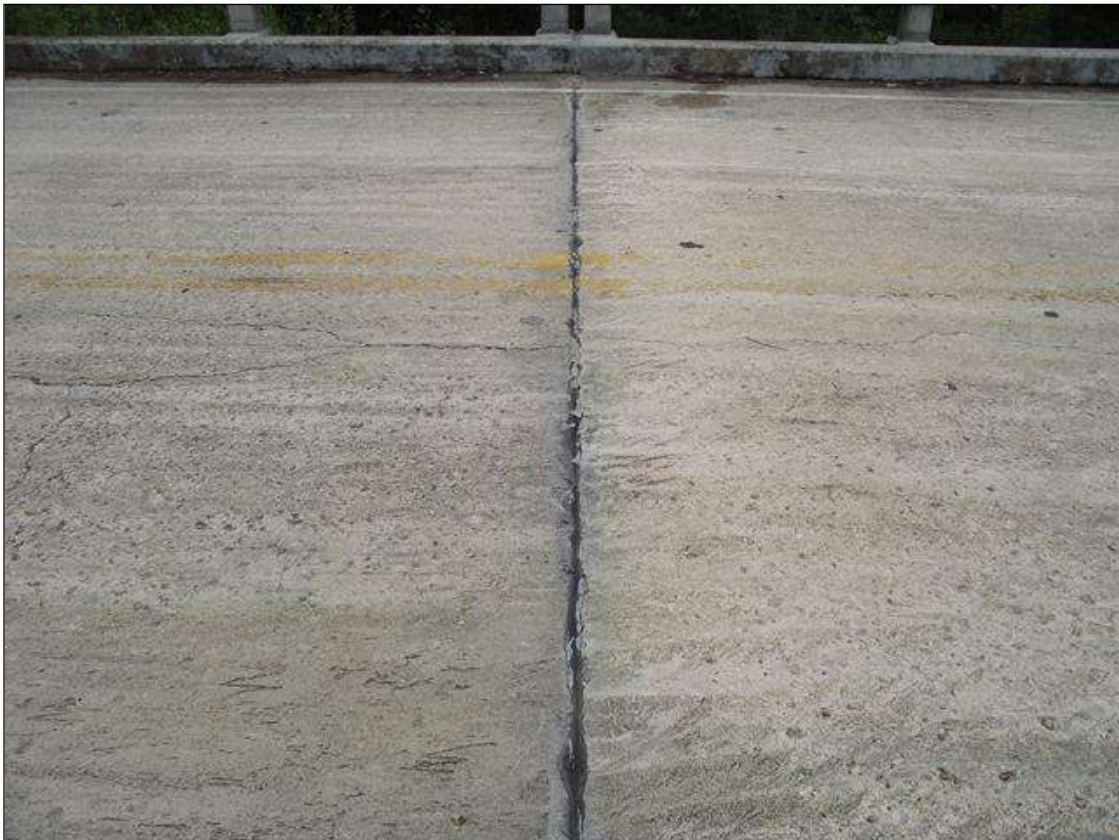
JOINT AT BENT 1
