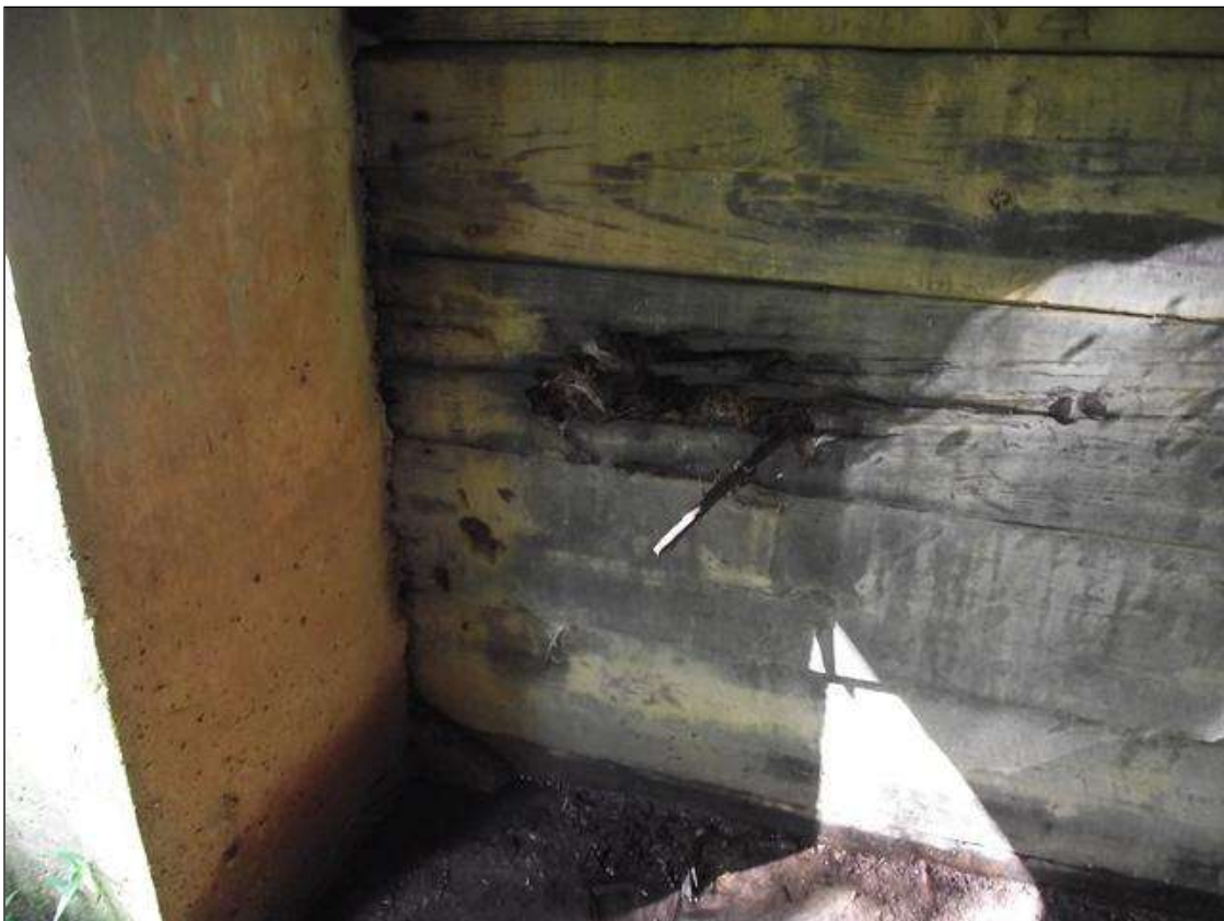
DECAY IN THE 3RD BULKHEAD BOARD FROM BOTTOM OF END BENT 1 CAP AND JUST TO THE LEFT OF PILE
